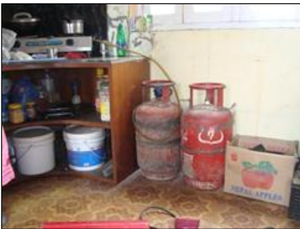
Fuel tanks affixed to the wall illustrate non-structural mitigation.
